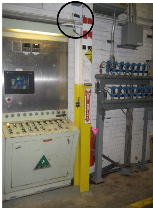
Figure 29: Example of Mesh Router deployed in a Heavy Industrial environment.
